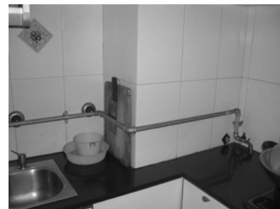
Fig. 16. Gas pipe in kitchen is exposed; becomes a convenient means to store knives and chopping board.
